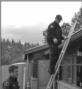
In between March storms, Capt Alan Lott (on ladder) cleans leaves & pine needles from IFPD station roof & gutters. Firefighter Dane Smith serves as his safety watch.
